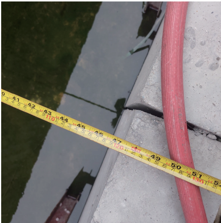
General View for point C, V11
